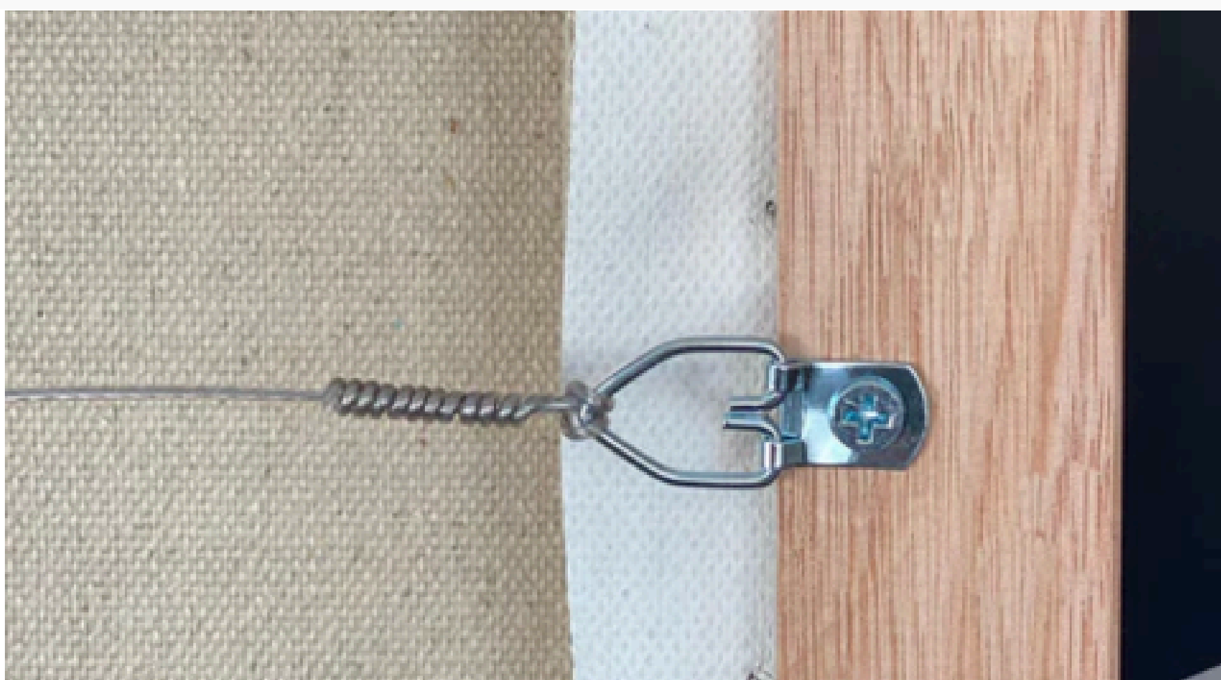
Figure iii - Successful D ring with wire installation
