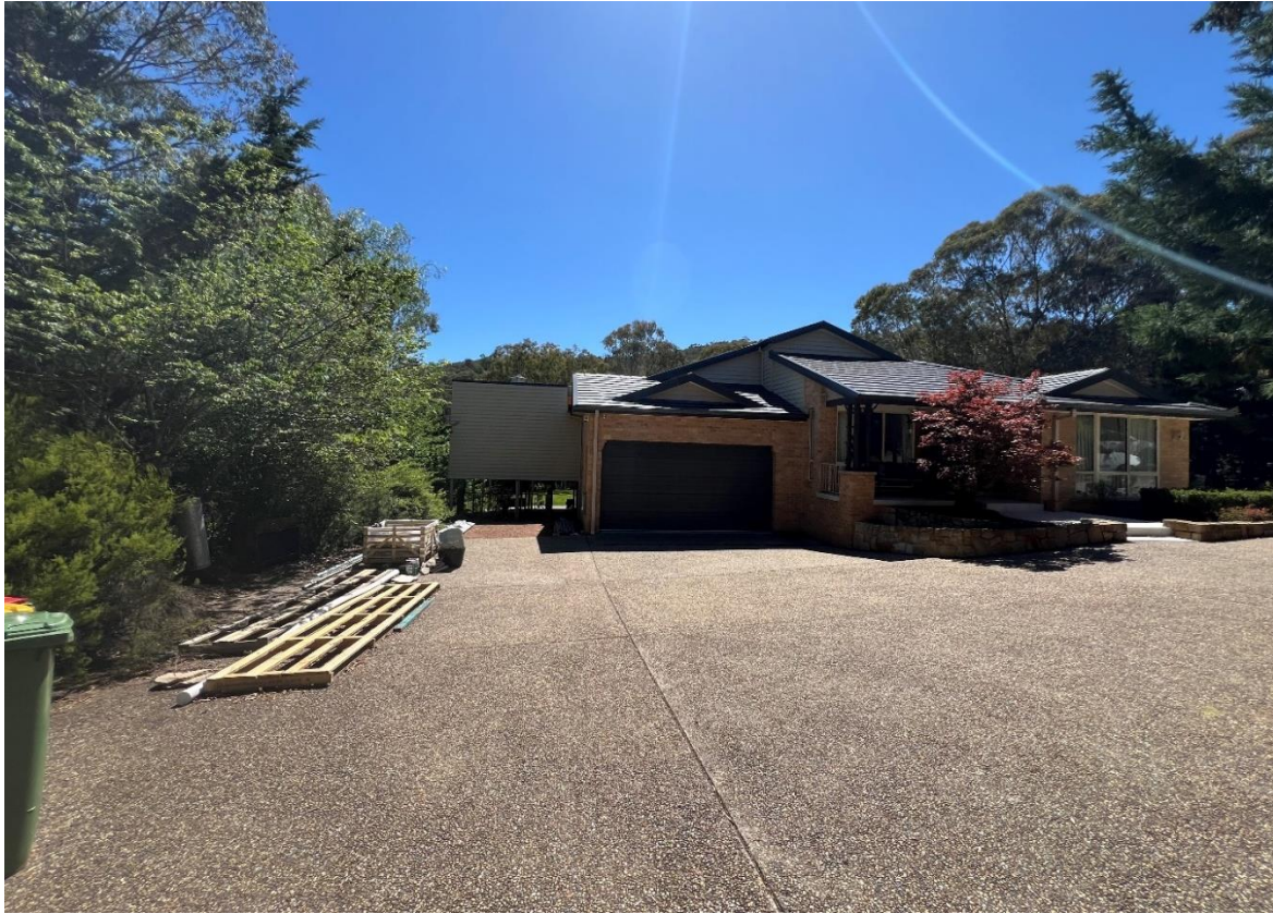
Figure 2: Front view of the existing dwelling
