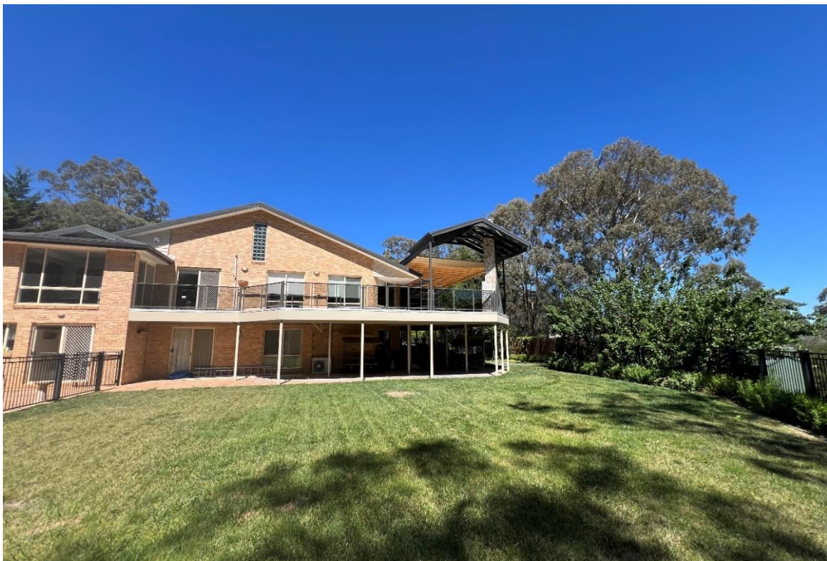
Figure 3: Rear view of the dwelling with the roof over deck at top-right side
