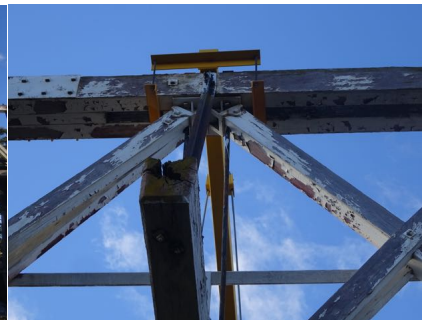
Photo 8: Close up of top of truss showing yellow cross brace.
