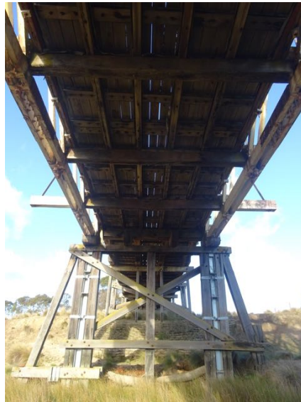
Photo 5: View of trestles and underside of road deck
