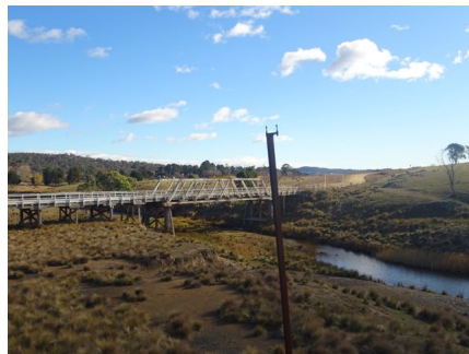
Photo 1: The bridge and its setting looking west
