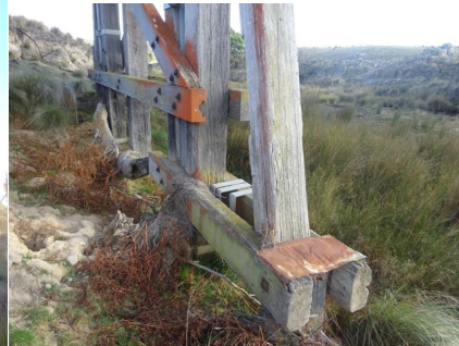
Photo 6: Detail of main trestle
