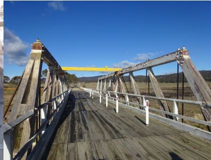
Photo 10: Road deck showing yellow steel cross brace and bounce back posts
