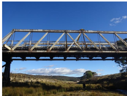
Photo 7: Main truss span, east side
