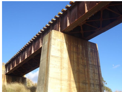
Photo 13: Concrete piers and steel girders
