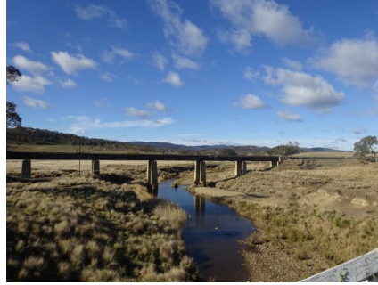
Photo 11: Railway bridge looking east bridges
