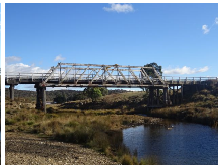
Photo 2: Close up of main truss span and support trestles
