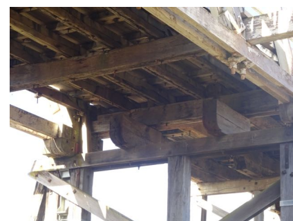
Photo 9: Detail of road deck support, showing simple curved corbelling.
