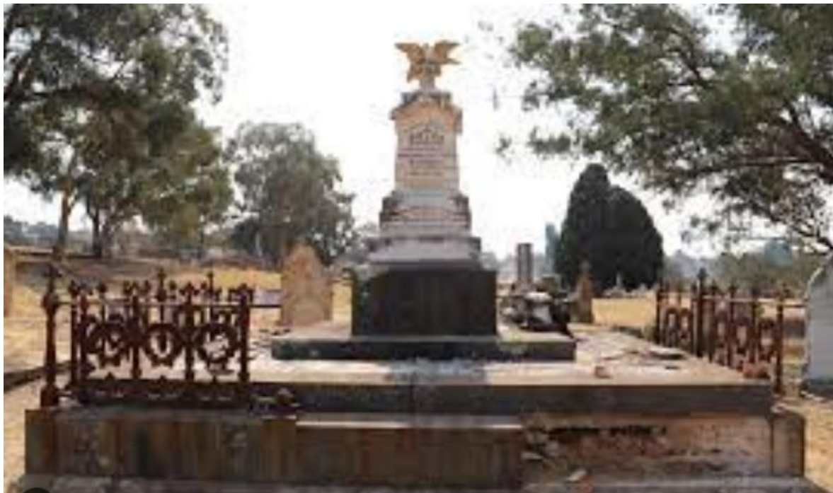
Example of a damaged memorial at the Queanbeyan Riverside Cemetery
