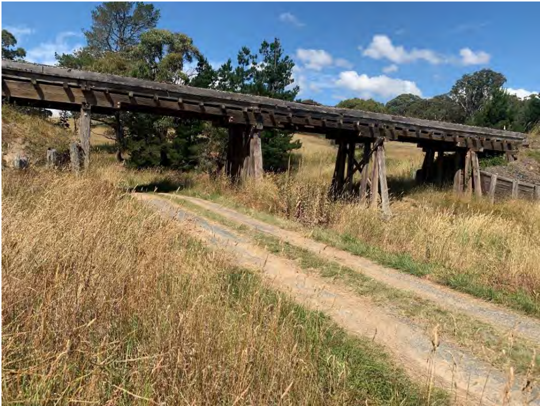
Figure 8-1: General view of Deep Creek Bridge from abutment 1 looking towards abutment 2. The timber bridge is 5 spans long and approximately 32 metres in length (Spans 1 & 5 – 4m and spans 2, 3 and 4 – 8m). Note span 2 passes over the road (4.2m Clearance) and span 3 passes over a creek 2m wide and 0.5m deep.
