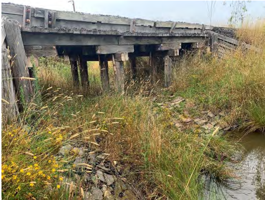
Figure 5-1: The top image shows a general view of the minor 10m Bridge from an abutment. The timber girder under bridge consists of 3 spans of 3.3m. Each bent consists of 4 driven timber piles and a single headstock. Headstocks are attached to the piles using a vertical steel bracket on either side. Note kerb support completely split vertically through middle.
