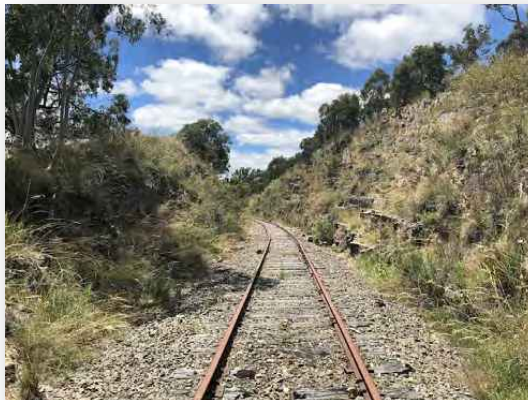
The old drains of the many cuttings along the proposed rail trail will require attention to ensure they still perform the task of clearing water from the cuttings.
