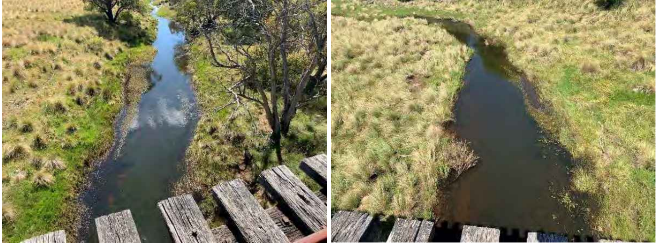
Figure 10-9: Left side image shows the view looking upstream and the right-side image shows the view downstream of the bridge of the edge of the open deck bridge.
