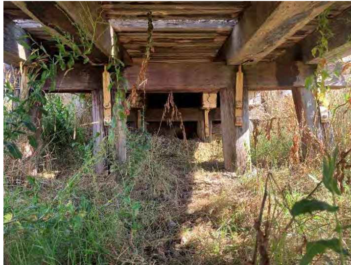
Figure 6-2: View of the typical timber pile bent configuration with each bent varying in height. The bent comprises of 4 driven piles a capsule (cap) and at bent 2 4 corbels located directly underneath girders. Overall, the timber bents were found to be in fair to poor condition. Note: large Wombat hole at abutment 2 between pile 2 and 3 and the significant amount of vegetation growth surrounding the substructure elements. Note that the use of horizontal bolts in the side plates have let to improved pile top condition. Also note the notches in the caps for the girders to drop into.
