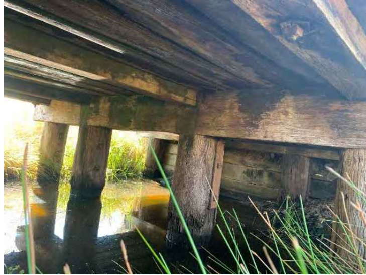
Figure 7-2: Shows the general configuration of the pile bents. Piles are approximately 1m high and in fair condition. Minor deterioration of sapwood is present at water level due to increased moisture content. Water stains and fungal growth present. Note: top plank in abutment sheeting has failed leading to erosion of backfill material.
