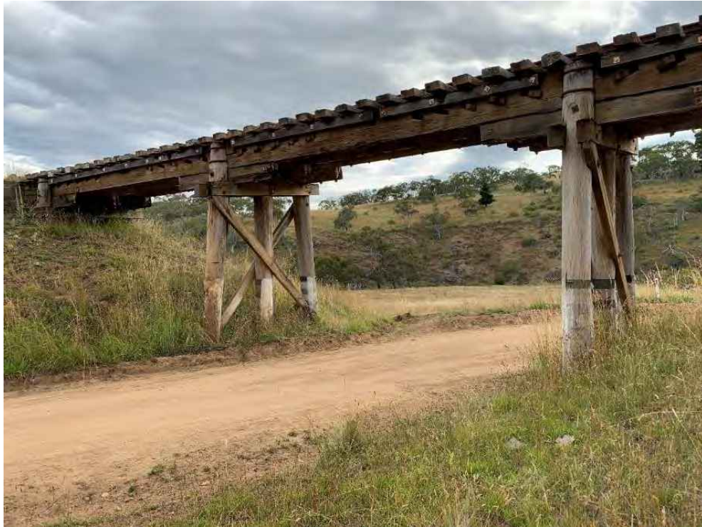
Figure 11-1: General view of Old Bombala Rd Bridge from abutment 1 looking towards abutment 2. The timber bridge is 3 spans long and approximately 22 metres in length (Sp1=7.8m, SP2=6.8m & SP3=6.6m). Note span 2 passes over the road (4.1m Clearance).
