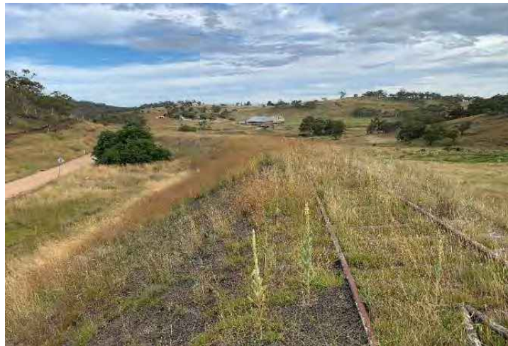
Figure 11-8: View of overgrown approach.
