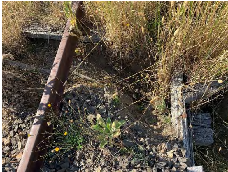
Figure 7-5: Top view of floorboards in the ballast tray at abutment. Large hole caused by abutment/ballast tray failure allowing significant erosion of ballast to occur.
