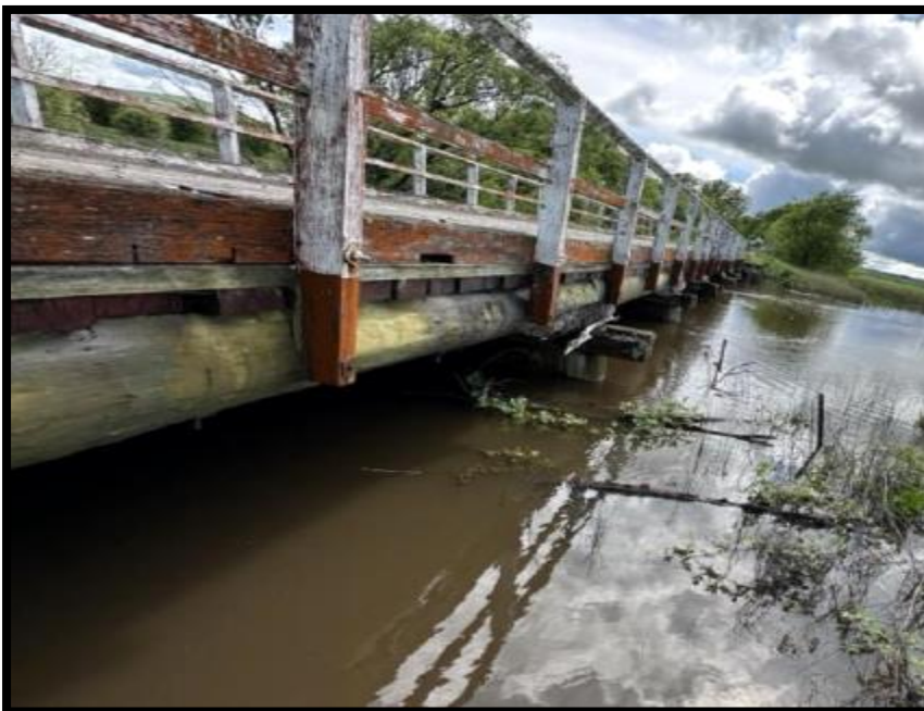
Figure 5 – bridge structure Bridge 2 (Source: Macrozamia Environmental Consulting)
