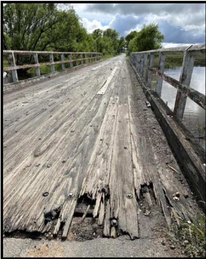
Figure 4 – Timber bridge deck Bridge 2 (source: Macrozamia Environmental Consulting)
