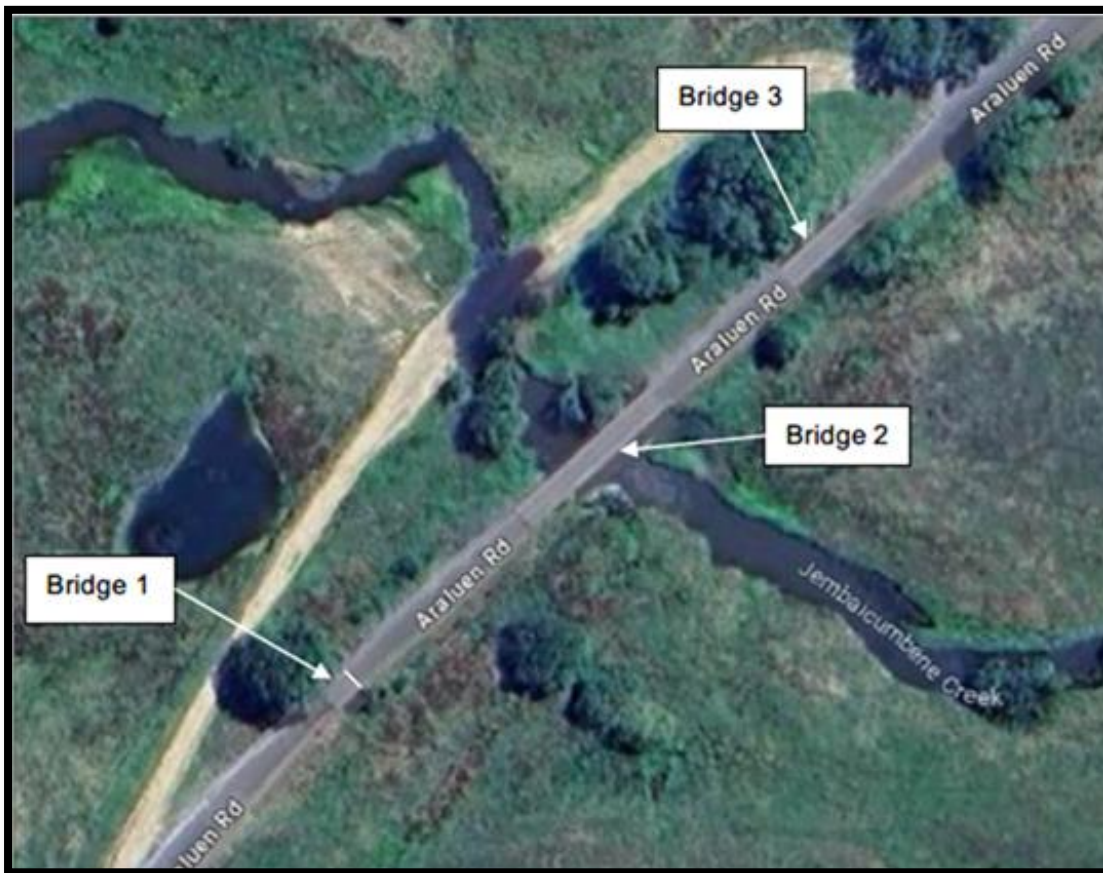
Figure 2 – Aerial image of bridge locations along Araluen Road
