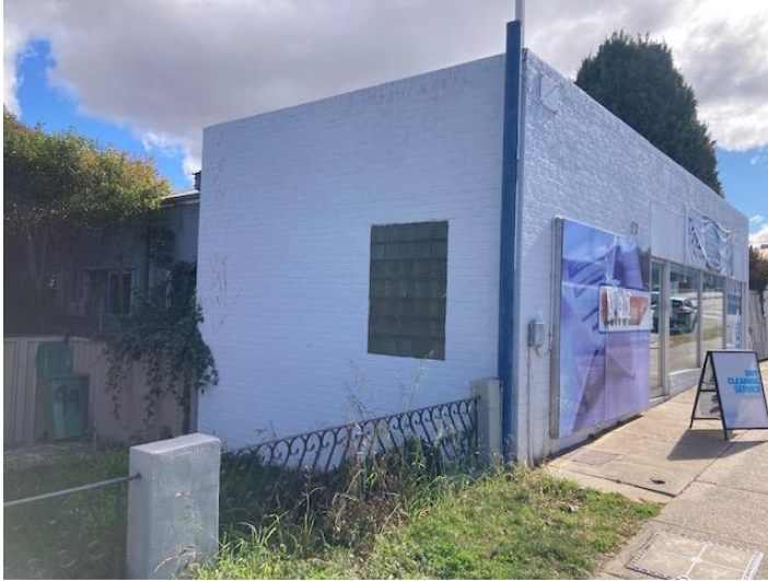
Figure 2 - Frontage to Crawford Street
