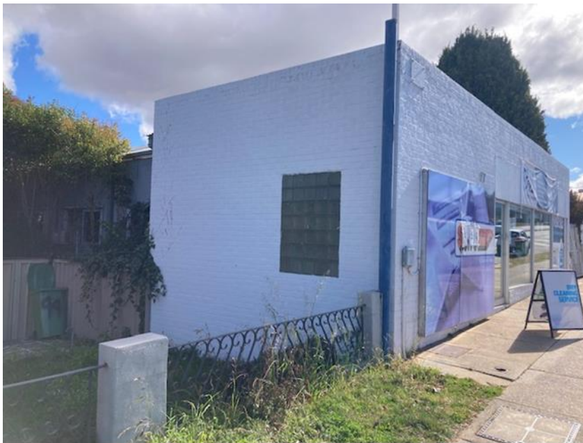
Figure 3 – Existing development fronting Crawford Street
