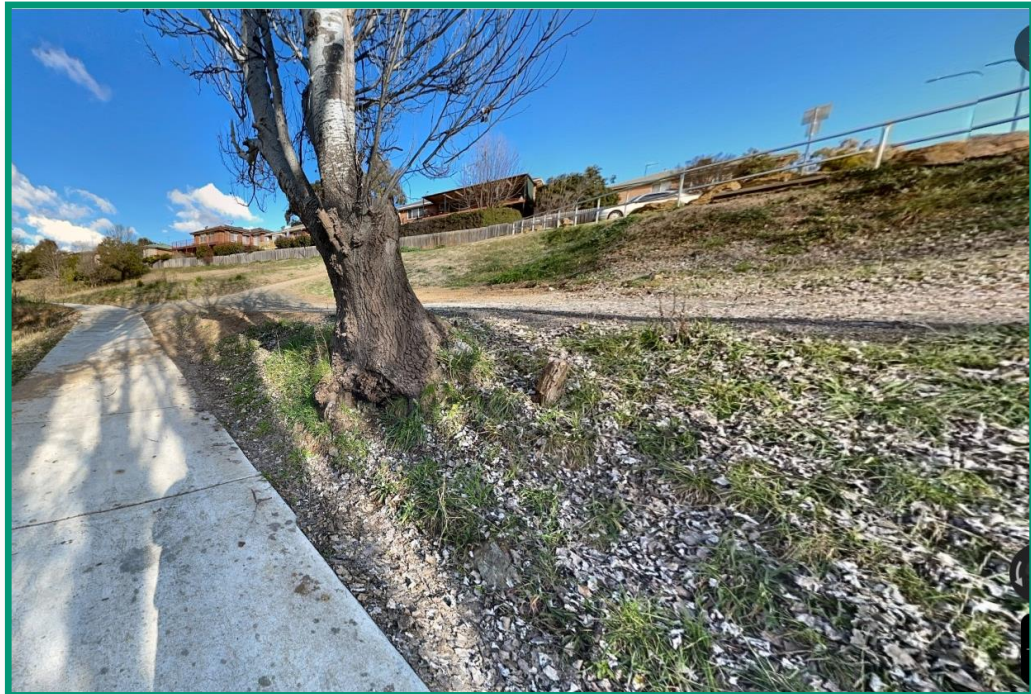
Figure 7: Google streetview image from footpath looking south east towards subject development source: Google maps
