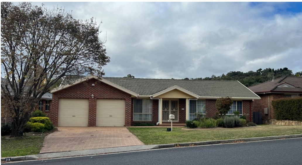
Figure 2: Front (south) view
