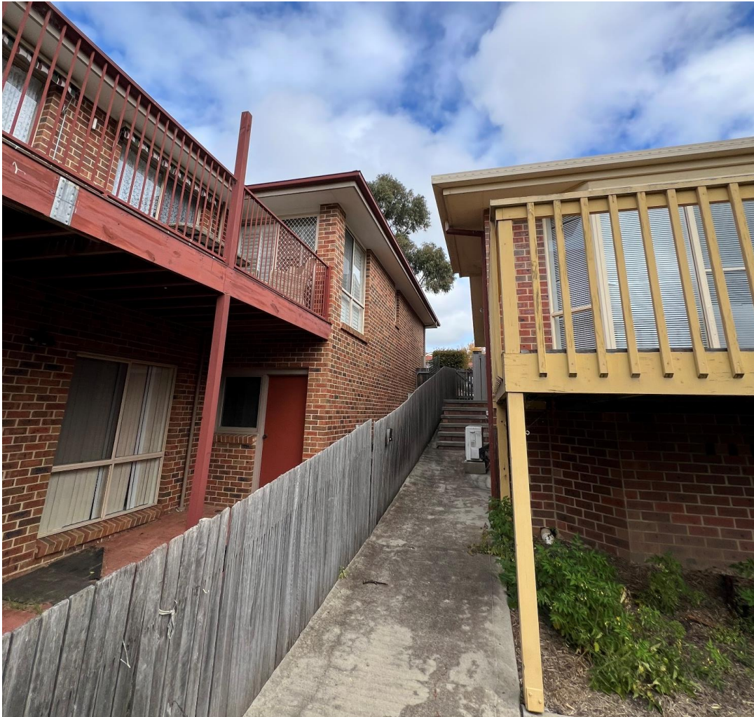
Figure 4: View along eastern boundary
