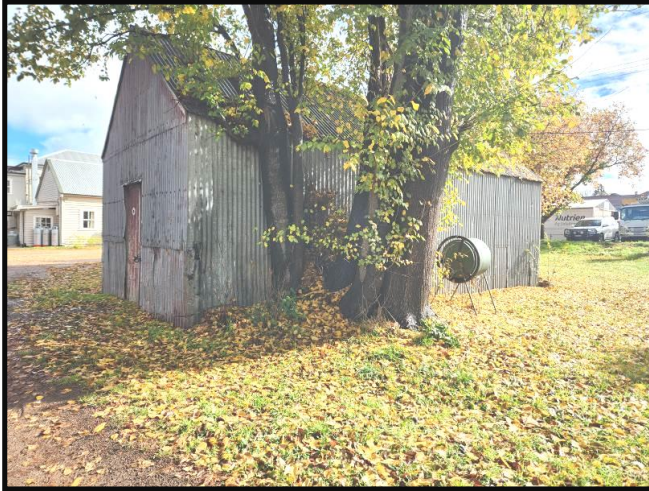
Photograph 3 Shows the East and South sides of the East Wing
