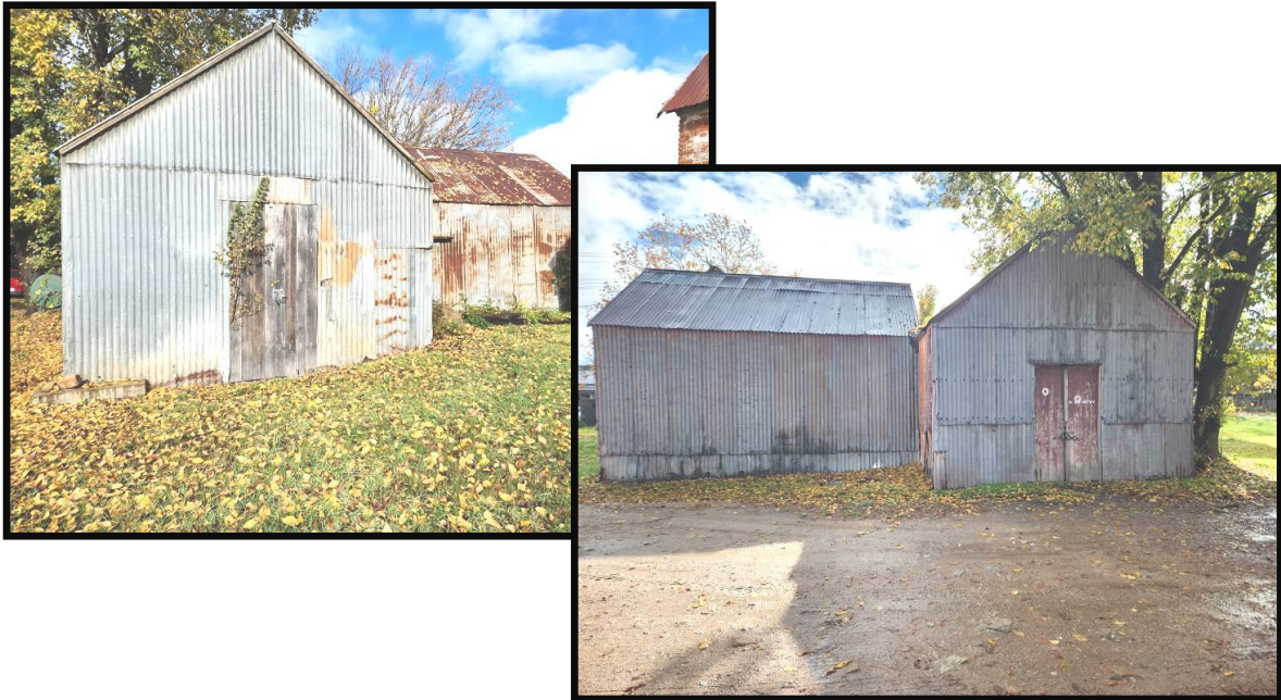
Front and rear of the sheds at rear of 119 Wallace Street Braidwood NSW
