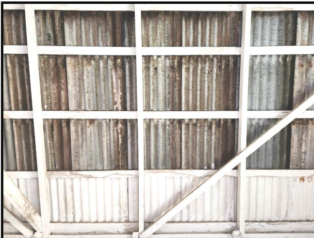
Photograph 6 Roof battens are 25mm thick & the span between rafters are approximately 920mm. Roof framing is a major structural component
