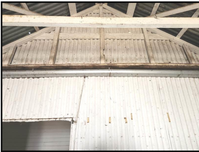
Photograph 25 Eave gutter to the East Wing, finished inside the West Wing
